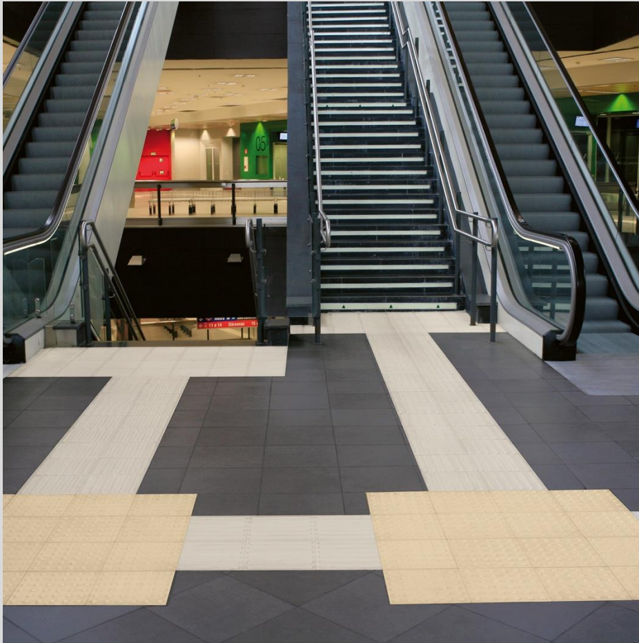
“PLAZA ELIPTICA” METRO STATION MADRID, SPAIN
