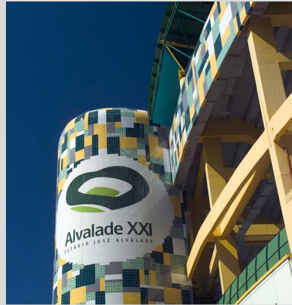
ALVALADE STADIUM LISBON, PORTUGAL
