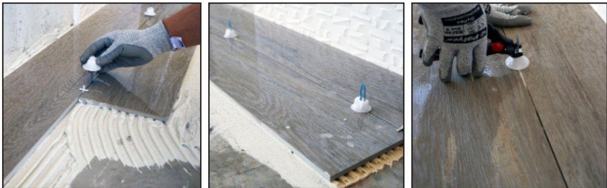
Fig. 27/28/29 Tile Level Quick, Rubi
