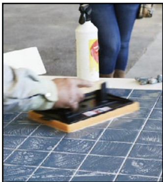
Fig.39 Clean the surface (with a sponge or damp cloth) and avoid using too much water, which will create spots in coloured grout. Make sure to remove all excess grout from the ceramic tiles.
