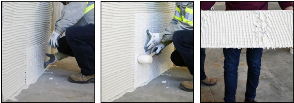
Fig.24 Next, tightly press the tile against the support surface to flatten the beads of adhesive cement, ensuring that it spreads so the area is fully covered. Fig.25 Tap the tile gently with a white rubber mallet to ensure that the back of the tile fully adheres to the support surface. Fig.26 Now and then, lift the tile to see that the bonding technique and the size of the trowel are suitable for the tile size and if the adhesive is being correctly transferred.
