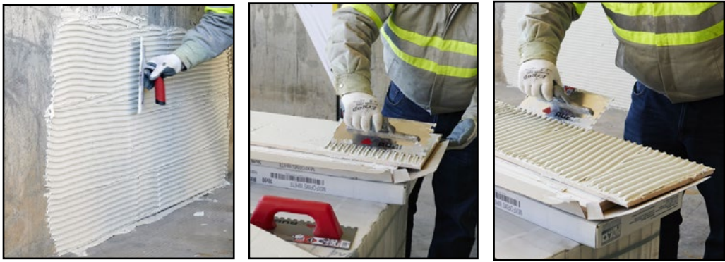
Fig. 21/22/23 Apply the adhesive cement in small sections (1m2 maximum) over the surface of the support, spreading it in thin, tight layers, using an appropriately chosen toothed trowel to remove excess water.
