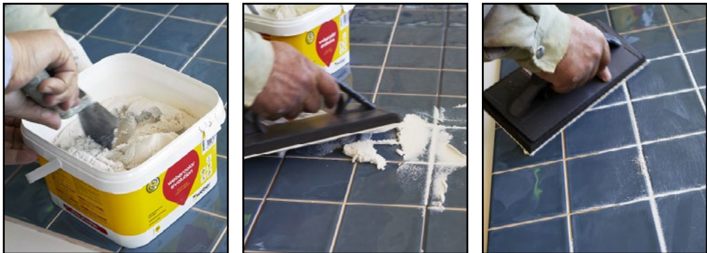
Fig.36/37/38 Apply the material diagonally over the joints, using a grout trowel. Spread the grout in the joints between the tiles uniformly to increase their durability.
