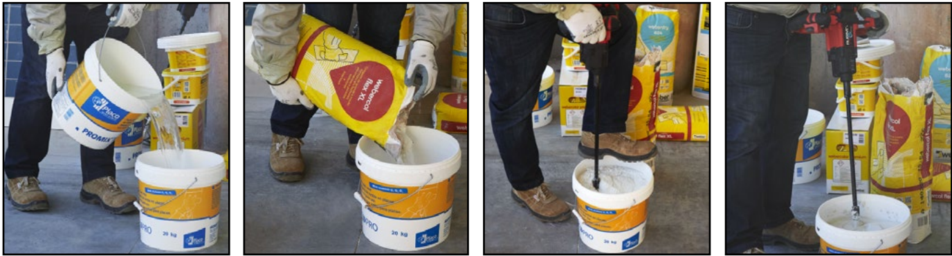
Fig. 17/18/19 Mix the adhesive cement with clean water using an electric low-speed mixer to obtain an homogeneous paste free of lumps. Let stand for two minutes and mix again.
