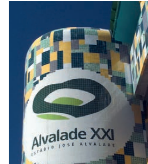
Estádio Alvalade XXI (Sporting Clube de Portugal) _ Arq. Tomás Taveira Alvalade XXI Stadium (Sporting Club of Lisbon) _ Tomás Taveira, architect
